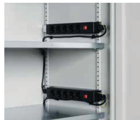
Side panel installation
