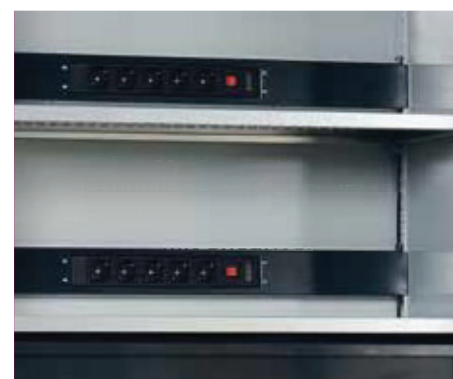
Rear panel installation
